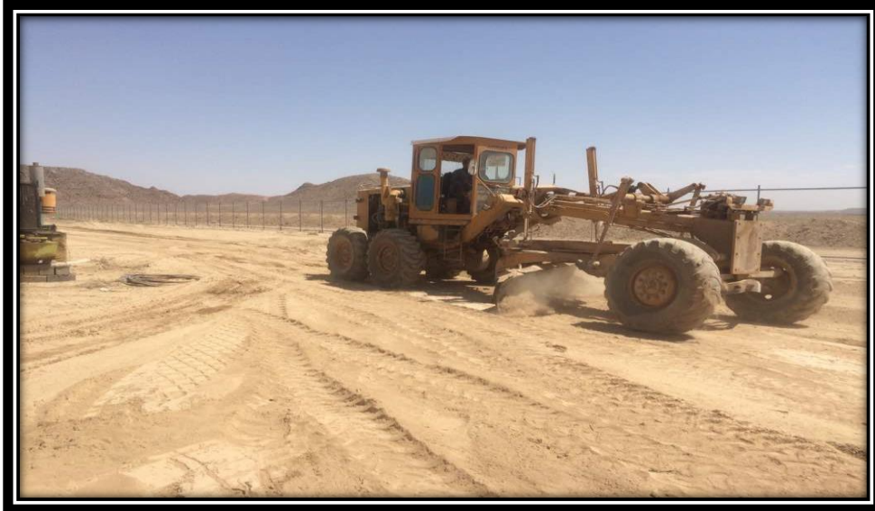
Leveling and adjustment operation by grader machine (Pouyan Gohar project)
